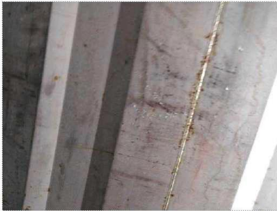
Superficial rust near the welding seam area, Refer to IICL General Guide for Container Cleaning, 3rd Ed.
