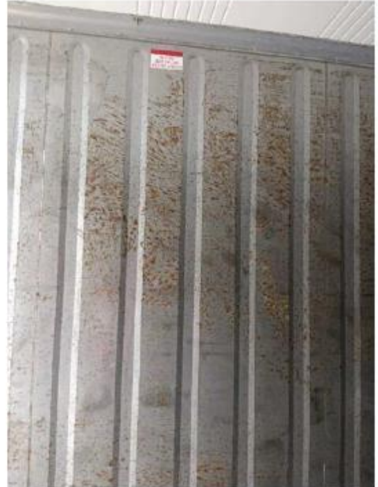
Contaminated panels showing rust/corrosion marks spread over large areas including weld seams, corrugated and flat surfaces. Above photos depict typical damage caused by contamination as result of chemical spraying. Repair required.
