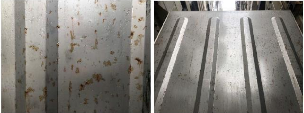
Rust/corrosion stains and pitting. Above photos depict typical damage resulting from contaminated panels after spraying with harmful chemicals. Repair required.
