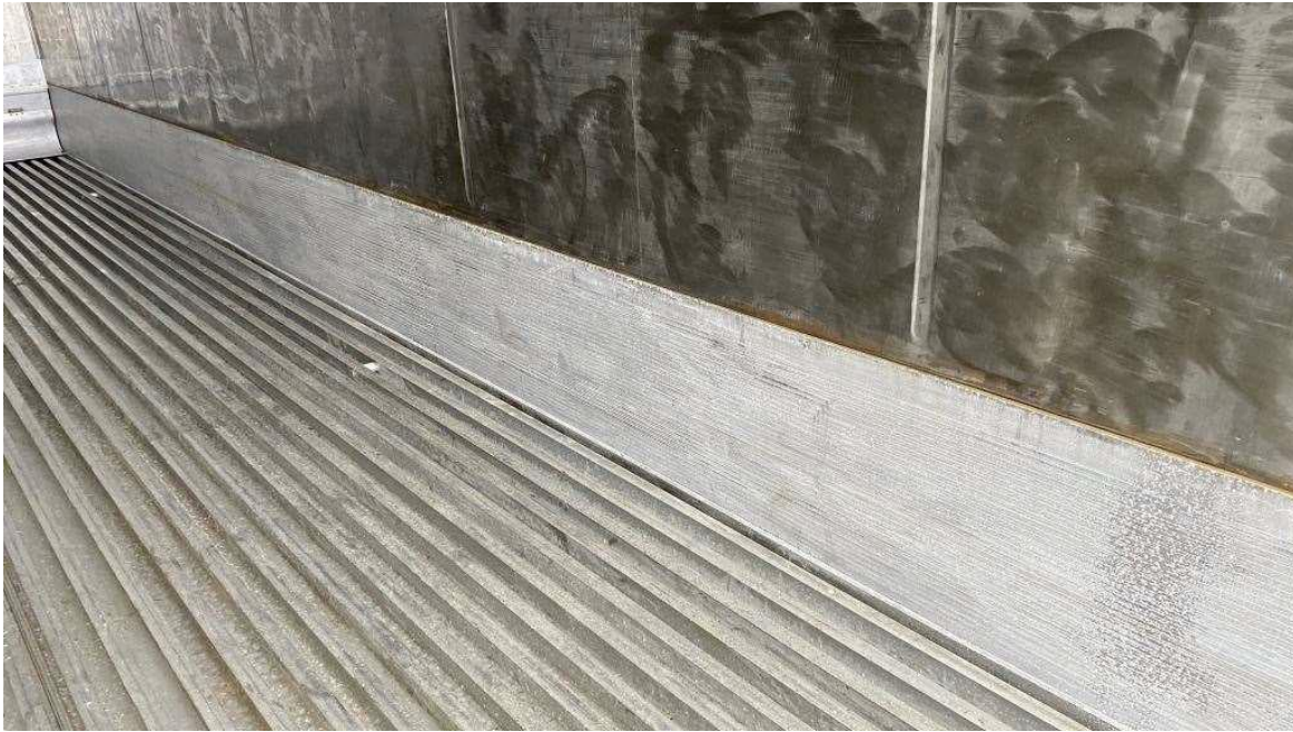
Contaminated scuff liner showing heavy oxidation and corrosion. Repair required.
