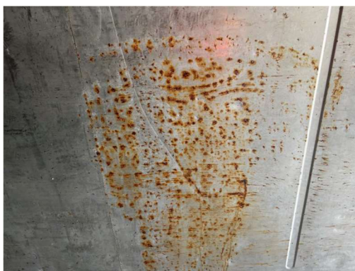
Contaminated HGSS panels showing corrosion as result of chemical spraying and scuff liner showing severe oxidation and corrosion process due to exposure to chemicals being sprayed. Repair required.
