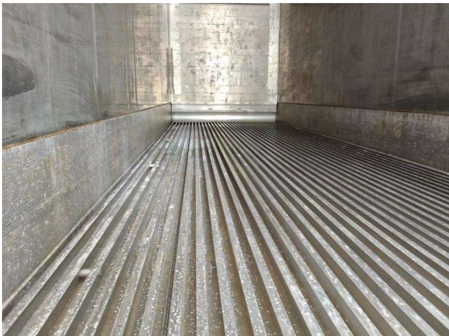
Panels, scuff liner and aluminium T-floor showing oxidation and corrosion as result of chemicals spraying. Repair required.
