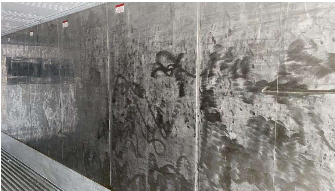
HGSS panels recently polished. Carefully look for existence of pitting, inspect machinery internal components.
