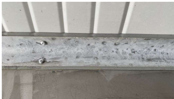
Contaminated interior aluminium coving showing oxidation and corrosion due to chemical spraying. Repair required.
