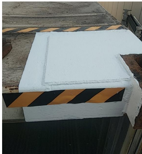
Rear Header and Corner Protection Plate repair sequence.
