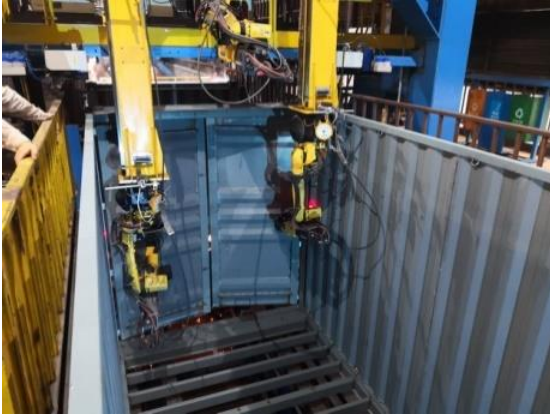
Stitch weld between side panels and corner posts
