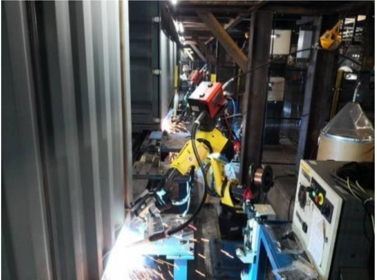
Robotic welding between side panels and bottom side rails.
